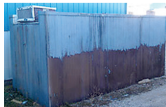
Enclosed walk-in freezer shed (to be removed)
