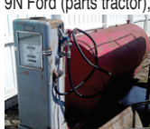
1000 gallon gas tank w/ pump
