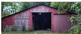
Barn (to be removed)
