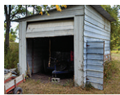
Lean to (to be removed)
