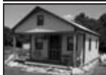
14' x 26' Cabin w/Porch & Loft
