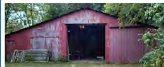
Barn (to be removed)
