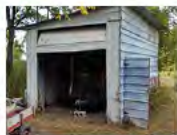
Lean to (to be removed)
